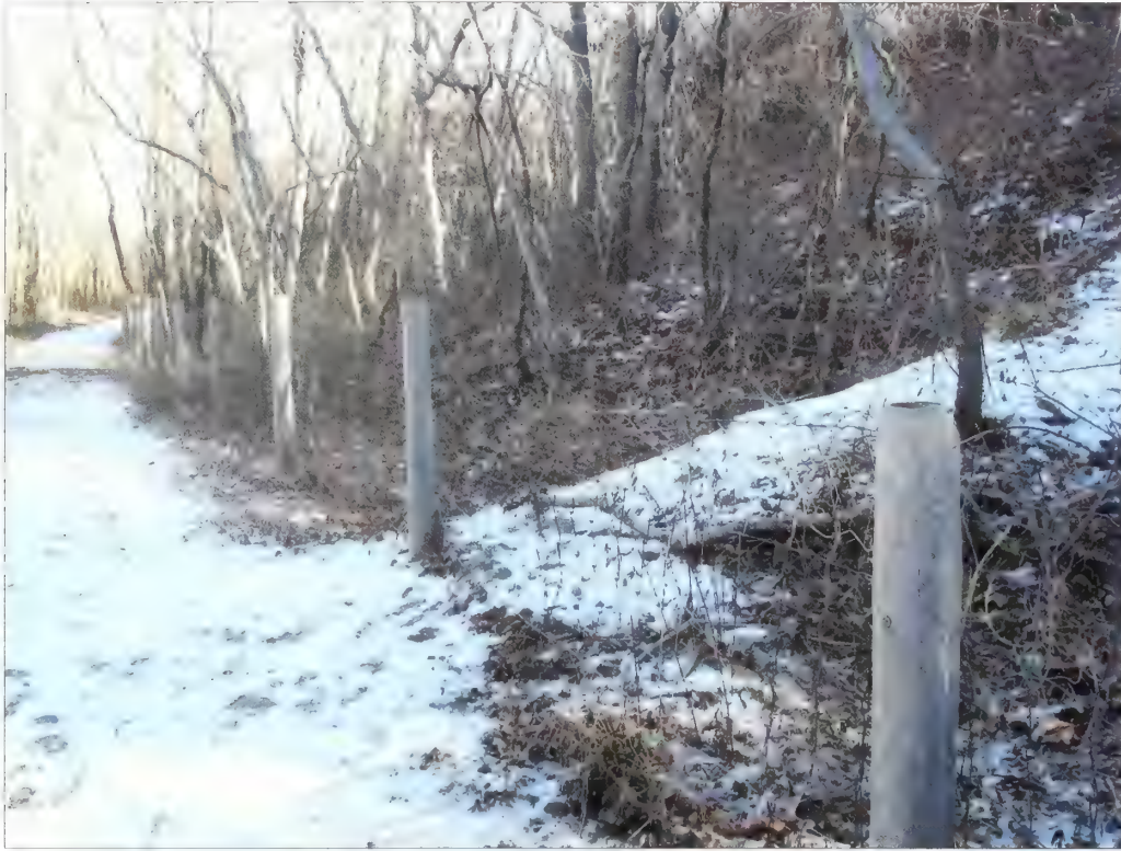
Figure 3.39. View looking northeast at toe of engineered earthwork, the Mortar Battery. East of the trail to the northwest and southwest emplacements, woven-wire mesh fencing is installed to discourage visitors from climbing up the engineered earthwork (Olmsted Center, January 2009).
